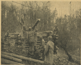
LOG HOUSES BEING BUILT NEAR FRONT
