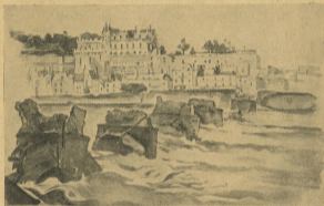
BRIDGES WERE BLOWN
