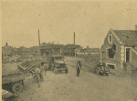
BRIDGE ON MAIN SUPPLY ROAD NEAR CARENTAN-JERRY SHELLED IT AT 10, 2, AND 4
