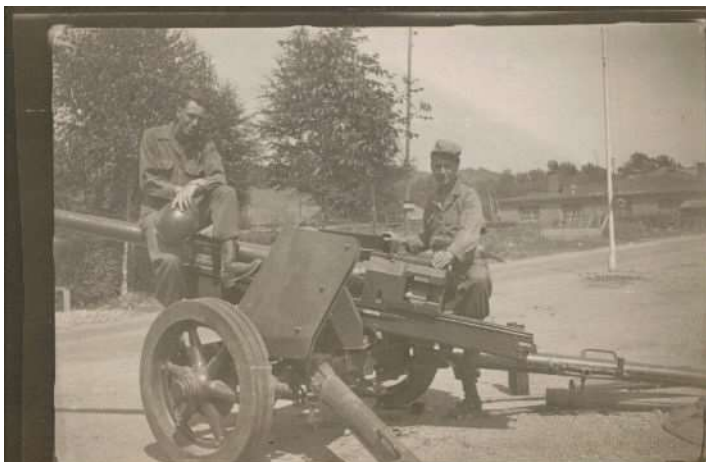
Photo, June 1945 in southern Germany, Wells and K D Austin
